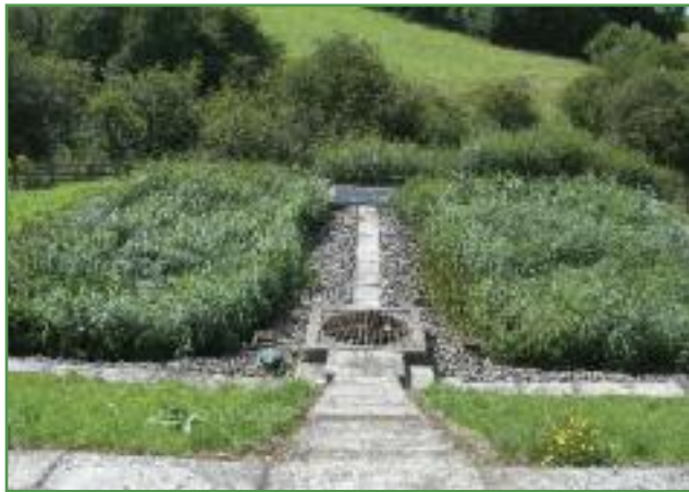
Common reeds being used to purify waste water, just outside the Eye Brook catchment at Lowesby sewage treatment works.
