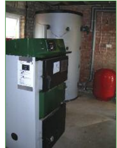
A modern high-tech woodfuel heating system for a local four bedroom house.
