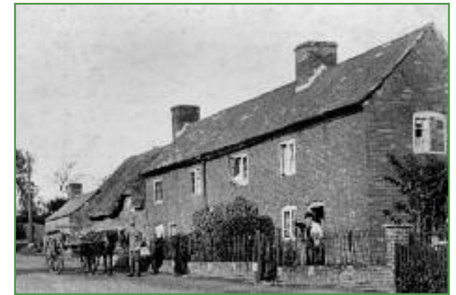
The baker's cart outside cottages at Littleworth, Belton. © June Lawton
