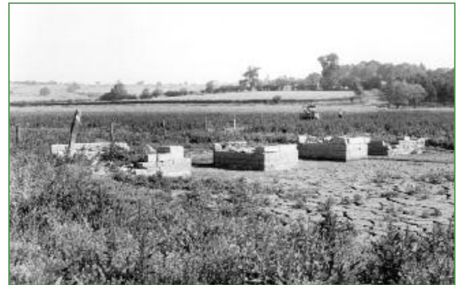
The foundations of Stoke Dry bridge revealed following drought in 1976.
