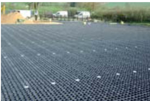
A permeable parking area is made from recycled silage wrap. The car park is sown with low-growing flowering herbage to attract insects and bees.
