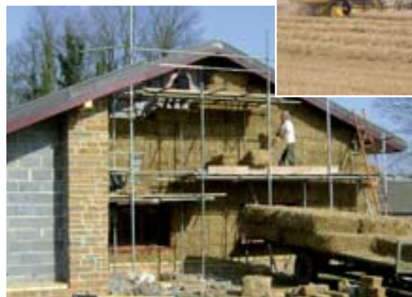
The wall insulation is constructed of straw bales made from the farm's own wheat straw.
