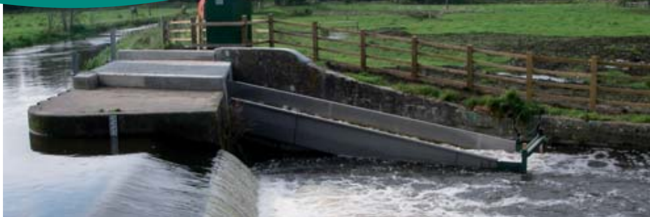
The installation of a fish pass at Loud's Mill, Dorchester, has benefited parr numbers. © Bill Beaumont/GWCT
