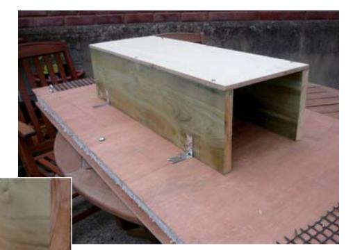
Attach the tunnel to the raft using right-angle brackets.
