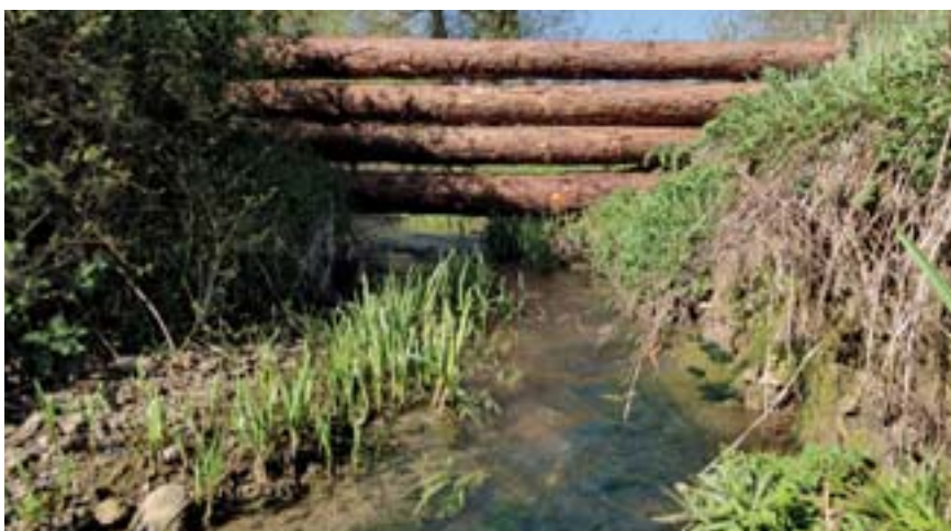
The creation of 28 permeable dams in the 1,000ha headwater resulted in a 19-24% reduction in peak flow at the base of the headwater.
